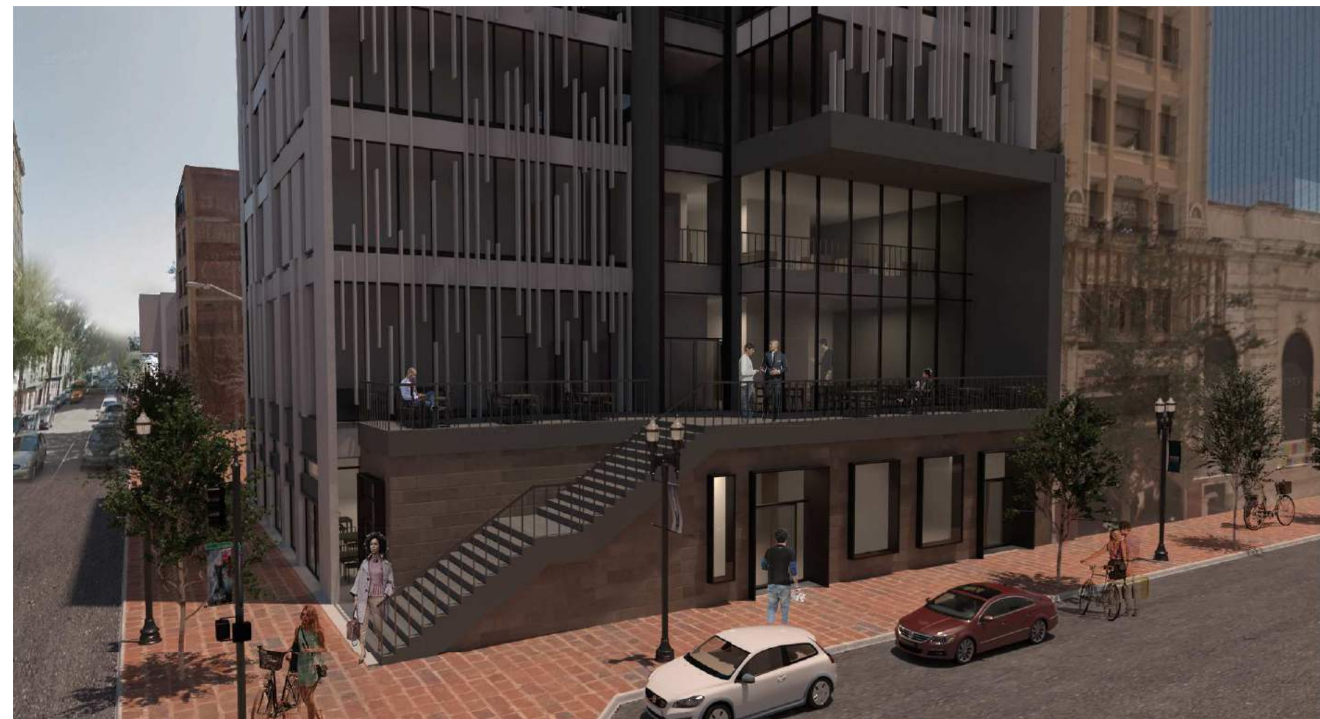
The Upper Deck Cafes and the Resident Entrance seen from the intersection of Adams and Laura st.
